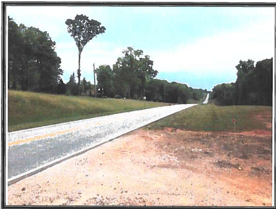
Street scene along SC Highway 11 Subject on right
